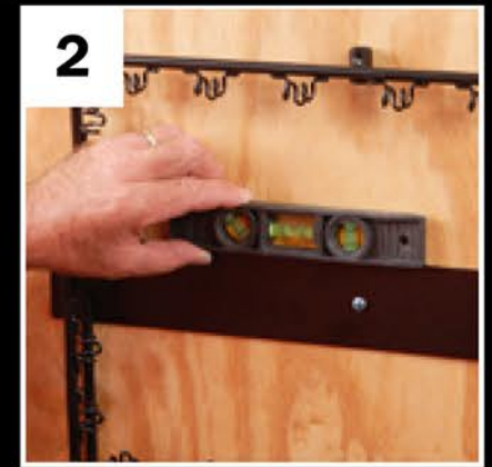
2 Use level to determine where the screws on either side of the plate should be placed and place a mark at these locations.
